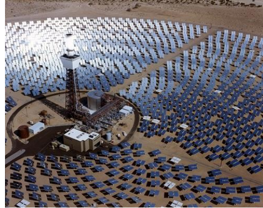
Fig. 5. CSP Power tower system requires water to cool down.
